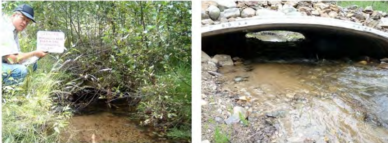
Figure 16. Photopoints and cross-sectional data related to the Granite Creek site Before (left) and after (right) construction. Left Photograph by Kathy Ramsey.
