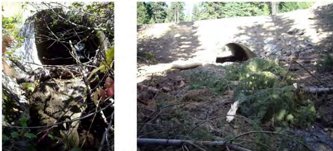
Figure 21. Photographs of the Bruin Creek Culvert Replacement site with photographs showing pre-implementation (left) and post-implementation (right) culverts at the lower end.
