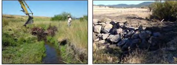
Figure 38. Photographs of the Fox Creek Channel Enhancement showing LWD installed in 2011 (left) and a finished 'plug' in 2012 (right).
