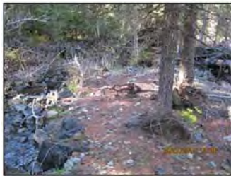
Figure 18. Photographs of the Bruin Creek culvert at the up-stream inlet (upper left), down stream outlet (upper right), and downstream blowout influenced channel (left). Pictures by Kathy Ramsey (UNF).
