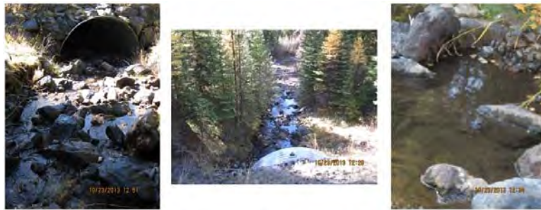
Figure 15. Photographs of the Battle Creek culvert at the up-stream inlet (left), down-stream outlet (right and center). Pictures by Kathy Ramsey (UNF).
