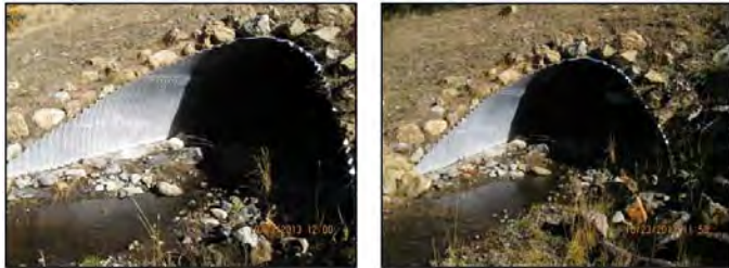
Figure 17. Photographs of the Bruin Creek Culvert Replacement site with photographs showing pre-implementation (left) and post-implementation (right) culverts at the lower end.
