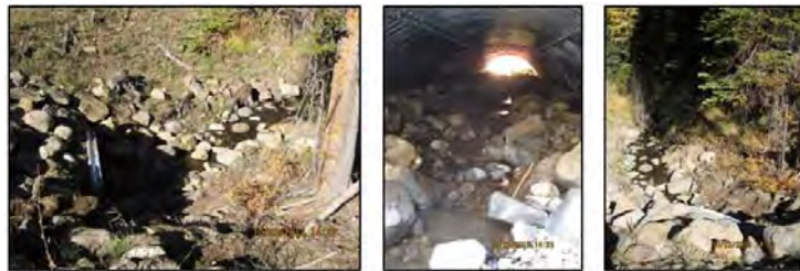
Figure 21. Photos of the new Upper Ten Cent Creek culvert at the upstream end (left), within the culvert (center), and lower end (right) during baseflow. Pictures by Kathy Ramsey (UNF).
