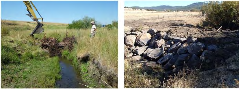
Figure 22. Photographs of the Fox Creek Channel Enhancement showing LWD installed in 2011 (left) and a finished 'plug' in 2012 (right).
