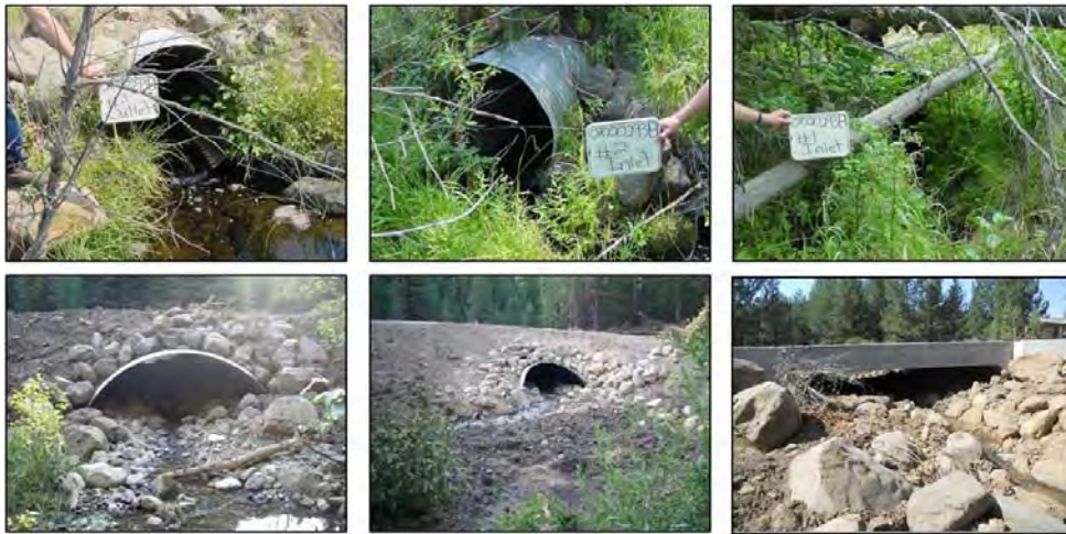
Figure 20. Photographs of the Ten Cent Creek culverts with pre-implementation on top and post-implementation below. Pictures are displayed from higher elevation (left) to lowest elevation (right).
