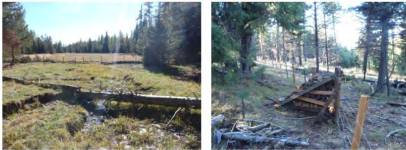
Figure 13. Photographs and cross-sectional data related to the Taylor Creek Fencing site showing the constructed fence (left) and a portion of the constructed fence (right). Photographs by Amy Charette.
