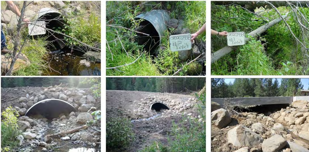
Figure 23. Photographs of the Ten Cent Creek culverts with pre-implementation on top and post-implementation below. Pictures are displayed from higher elevation (left) to lowest elevation (right).
