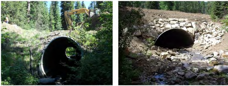
Figure 15. Photopoints and cross-sectional data related to the Battle Creek site Before (left) and after (right) construction.
